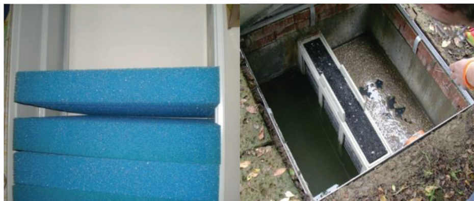
Figure 2. Photographs showing the finishing filter, consisting of a filter holder and a sponge, before and after use
